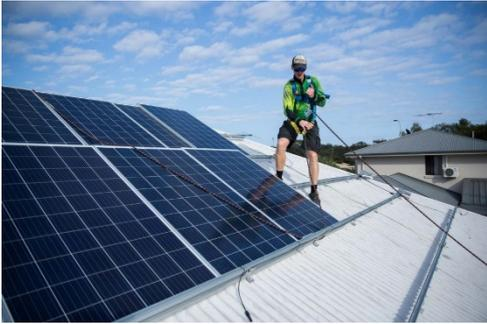
Figure 4 Incorrect use of rope systems can lead to massively increased risks
