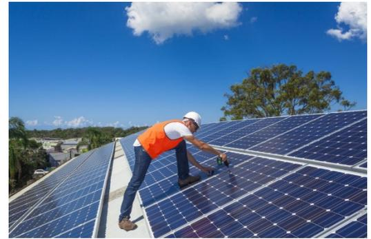
Figure 1 Incorrect safety provision for maintenance workers is wide spread
