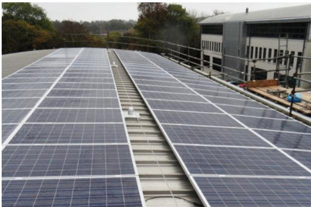
Figure 6 Panels and Lifelines positioned for ease of access
