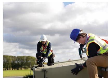
Figure 3 Roof Repairs using a horizontal lifeline and suitable PPE
