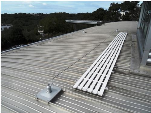
Figure 1 Walkway and Lifeline for window and gutter access
