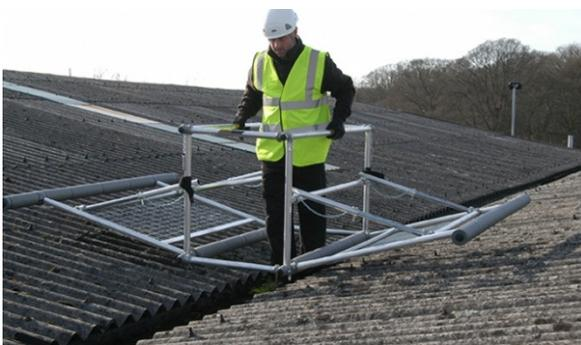
Figure 6 Mobile Barrier systems employed to allow gutter access for maintenance
