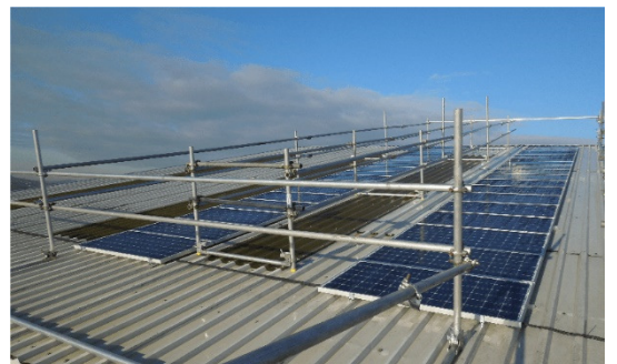
Figure 3 Scaffold provides safe access in some areas, but is costly
