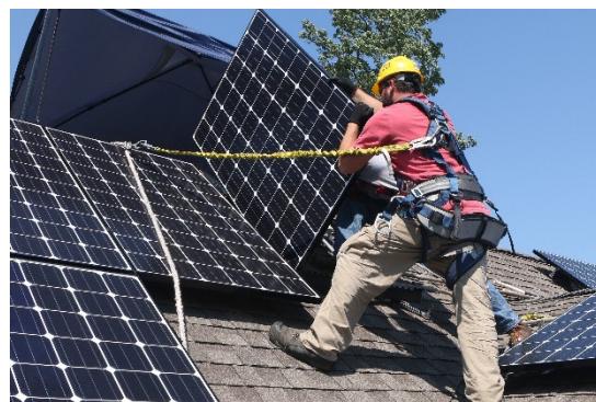
Figure 5 Use of fixed length lanyards reduces risk
