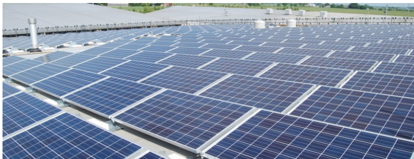
Figure 2 Designed for maximum output means minimal access and safety
