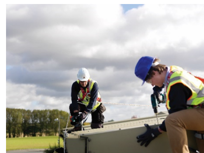
Figure 3 Roof Repairs using a horizontal lifeline and suitable PPE
